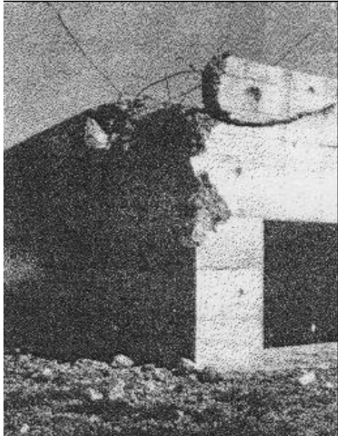
Fig 15 Damage to corner of target caused by Bomb No 3
